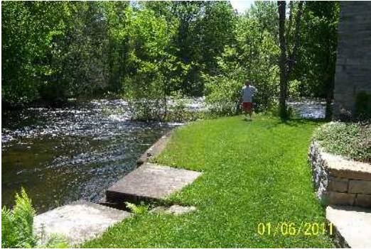
McCabe Grist Mill Shore Foundation & Island Sluice
